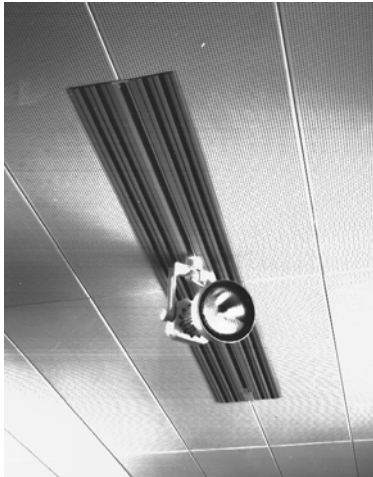
LTG linear diffusers type LDB 12/8/2/12 with a lamp rail integrated in the air distribution box.
