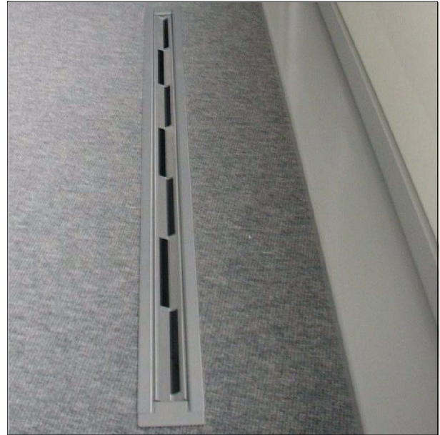
Floor-mounted linear diffuser type LDU 30/1/..., installed
