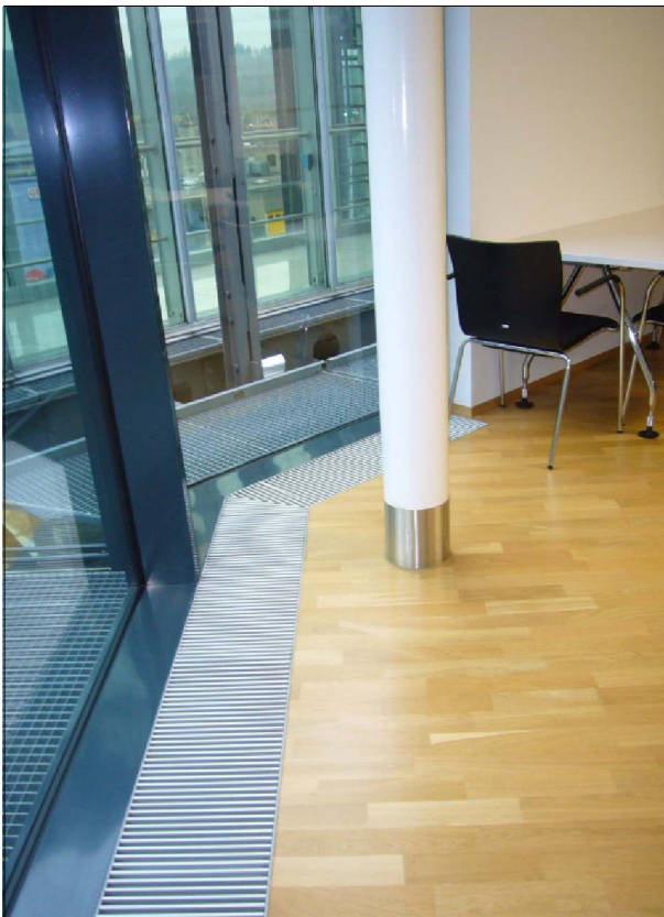
Installation example, with LTG aluminum roller grille
